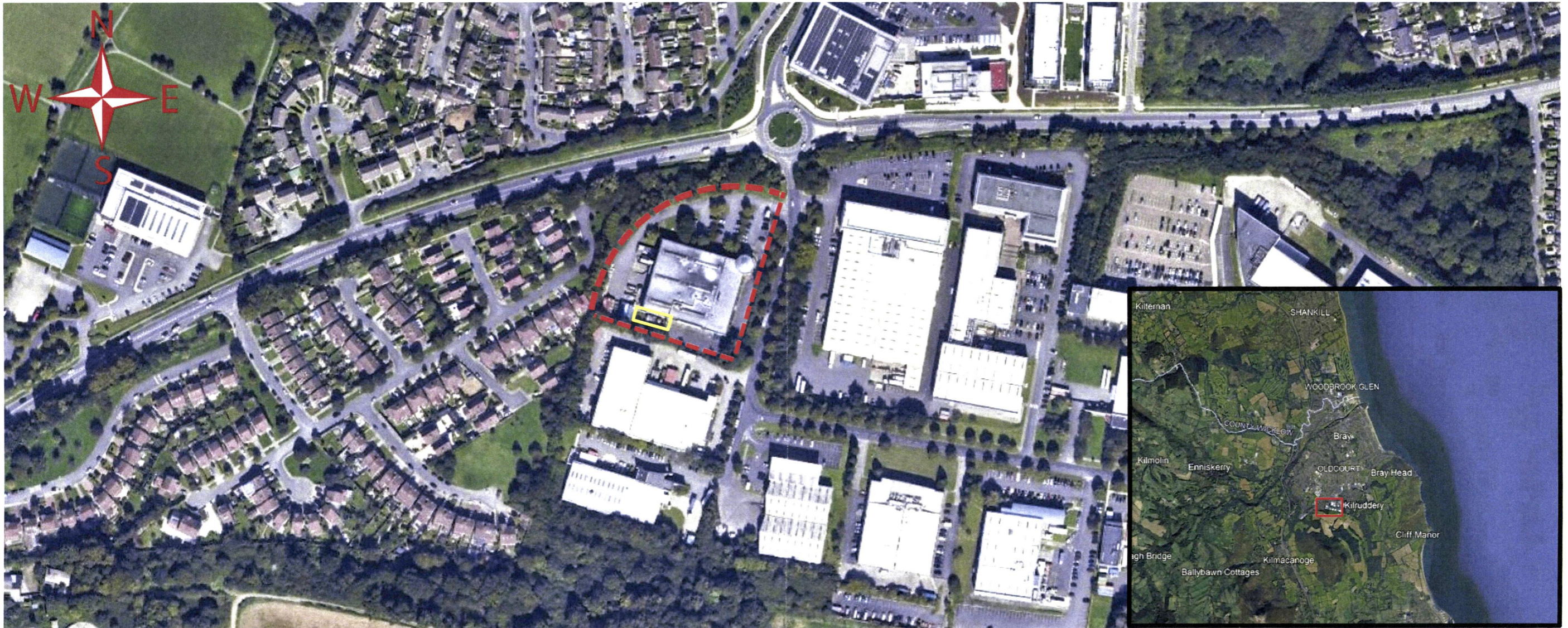
Figure 1: Aerial photograph showing Alert Packaging location in Bray, County Wicklow. Red dashed line outlines Alert Packaging property perimeter. Yellow solid line outlines abatement system area.
